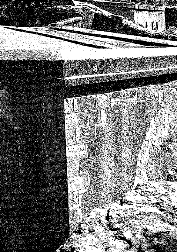
A corner of Biet Mariam reconstructed with modern brick and cement.
