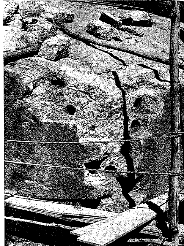
Same corner after removal of incongruous additions but before restoration to monolithic form and appearance.
