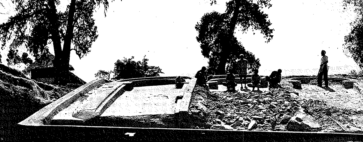
The heavy layer of grey cement being carefully chipped away from the roof of Medani Alem to expose the original monolithic surface.
